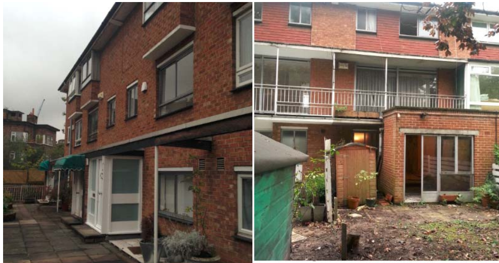
Figure 28 Rear and front of 14 Avenue Road
