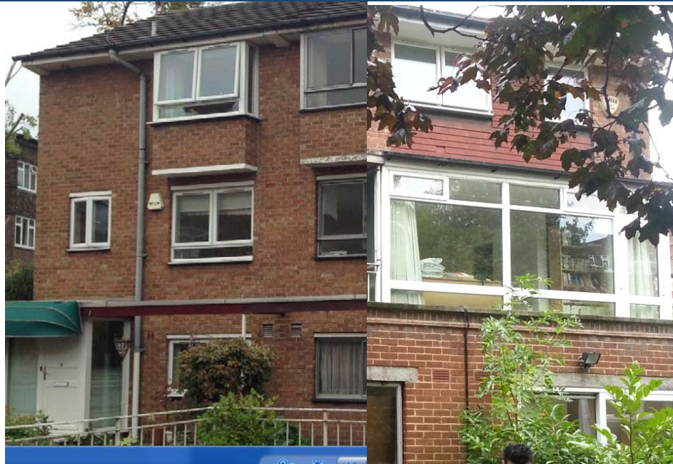
Figure 30 14f Avenue road front /rear of the building
