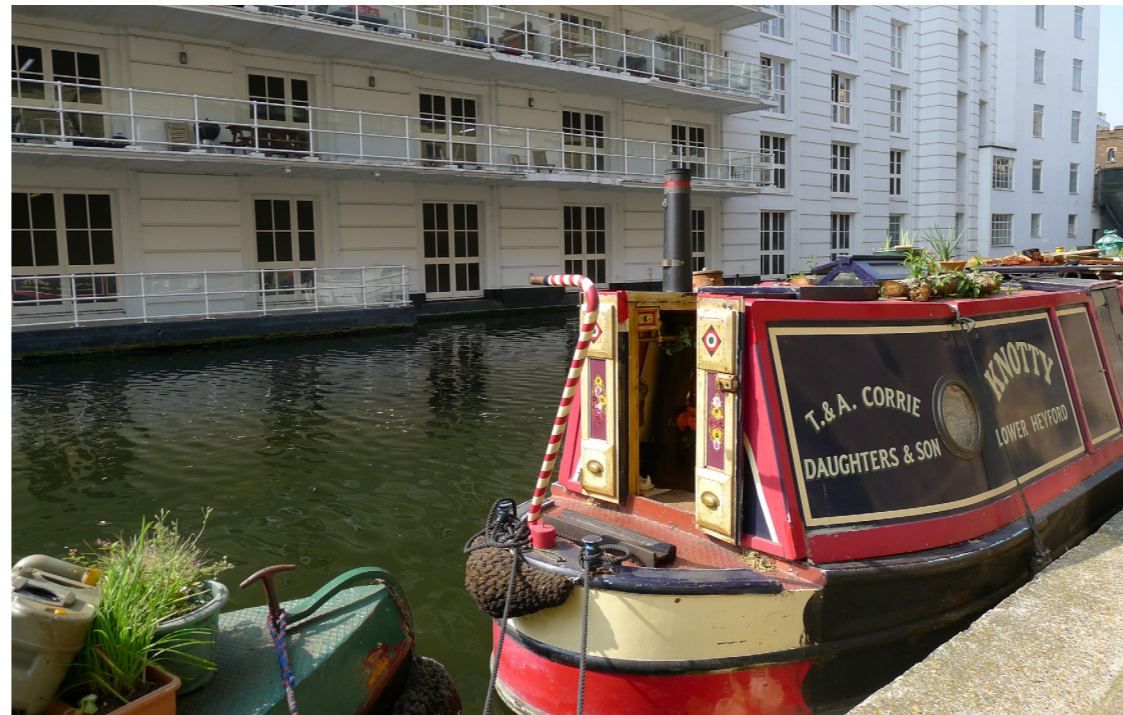
Balconies protruding over canal
