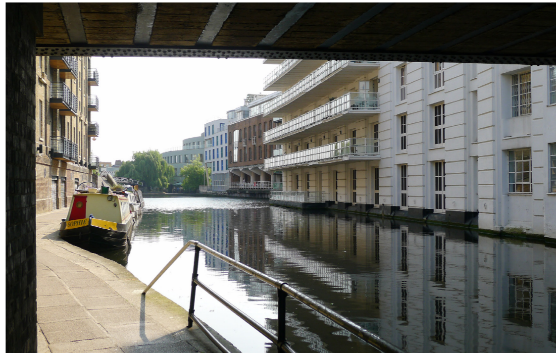
Heavy masonry piers of Gilbey House giving vertical character to canalside buildings
