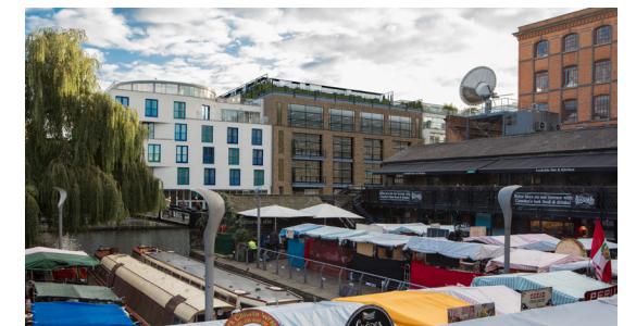
Previously consented view 03: from the Stables Market
