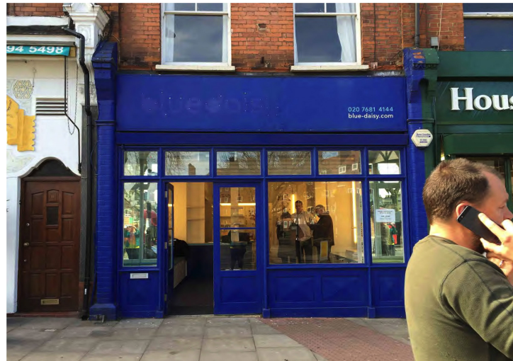
EXISTING FRONT ELEVATION PHOTO SCALE NTS
