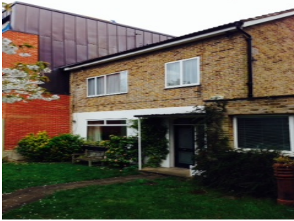
FRONT VIEW – VIEW FROM THE INSIDE OF THE PROPERTY
