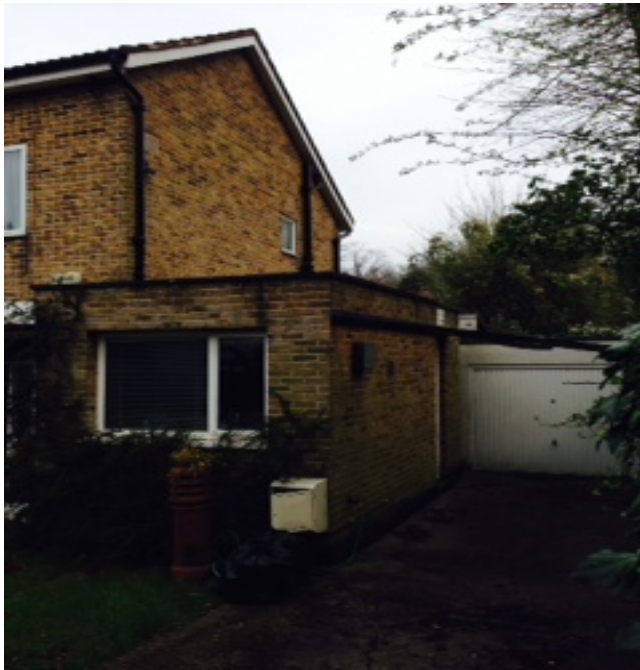
FRONT VIEW – VIEW FROM THE INSIDE OF THE PROPERTY
