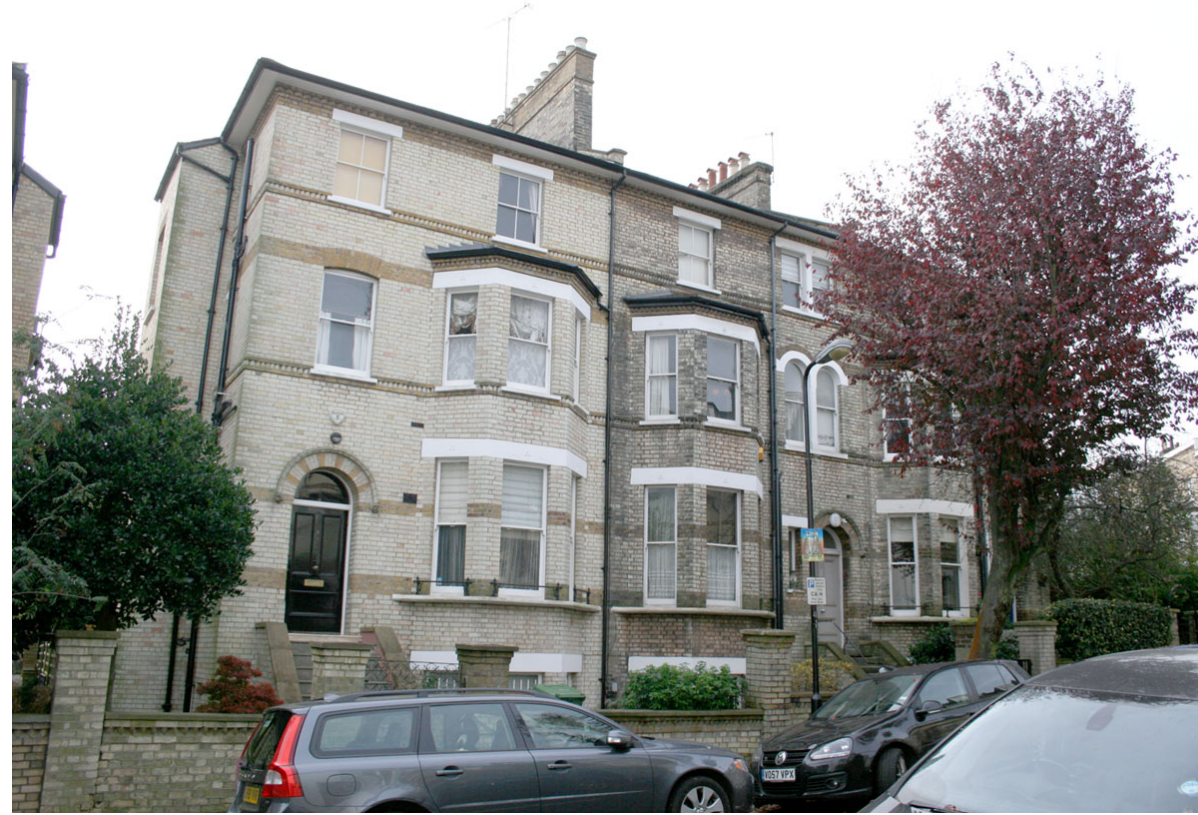
No.1, 2 & 3 Gayton Crescent.
