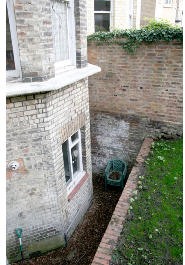
Rear Patio at Lower Ground Floor of No.2 Gayton Crescent.
