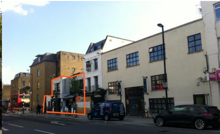
Street view from the north (close proximity)
