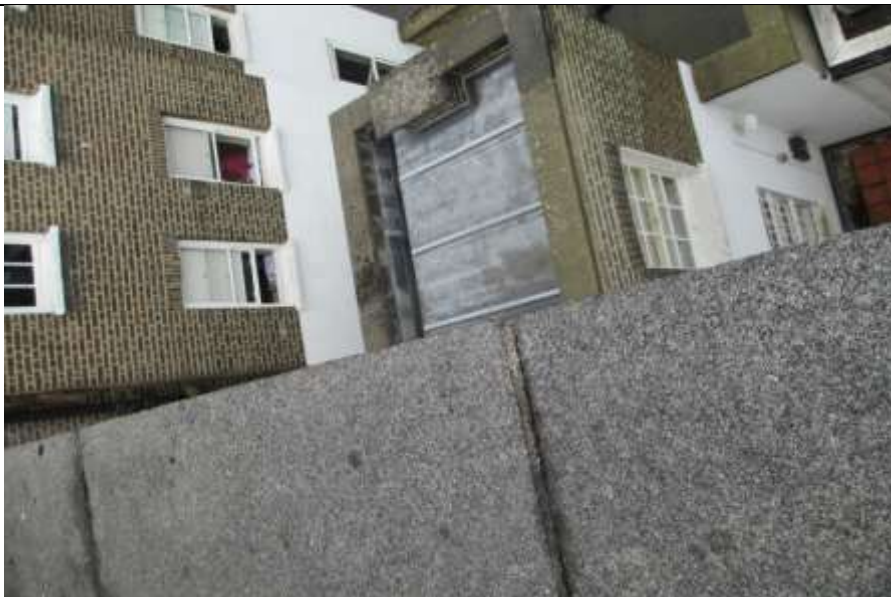
2. Parapet around flat roof to rear addition.
