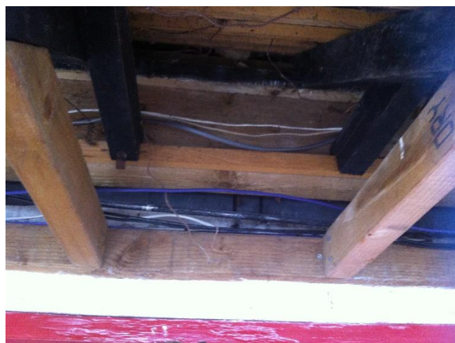
Underside of canopy to be removed
