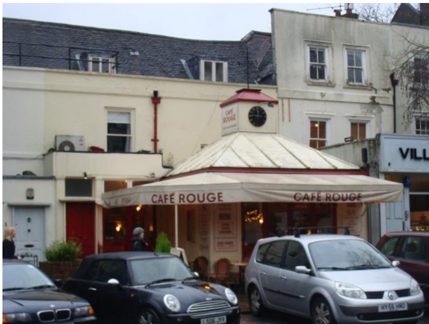
Existing front extension
