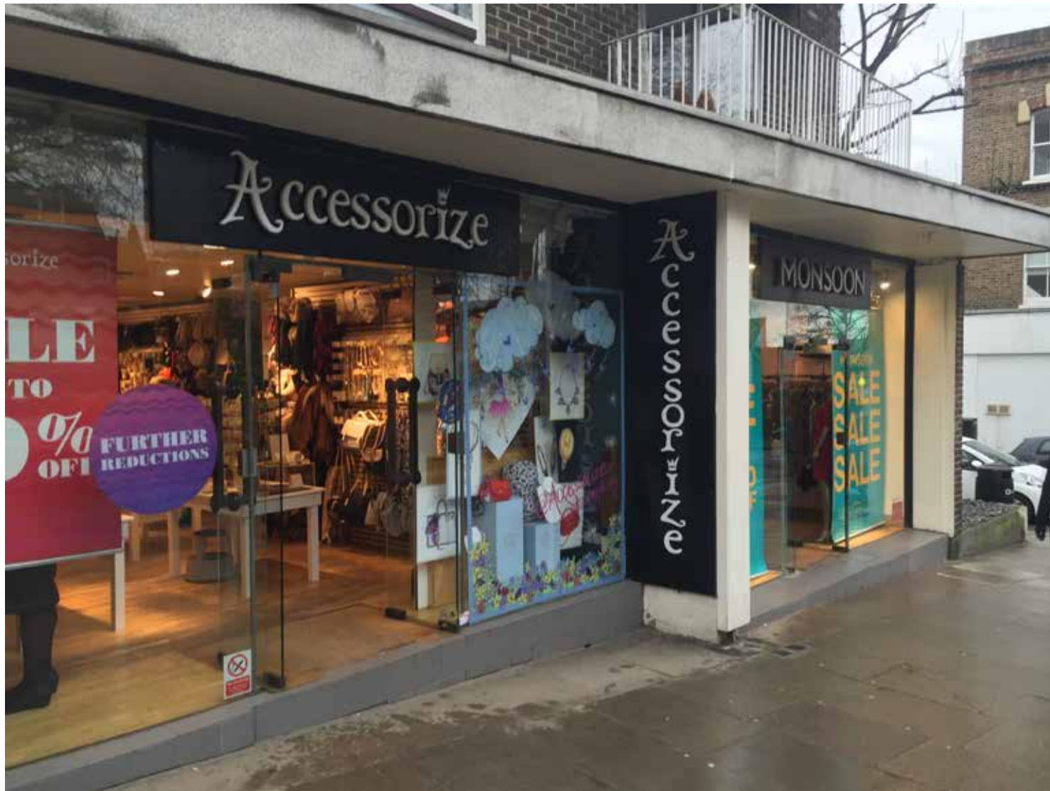
No's 1b & 1c Hampstead High Street. Photograph from March 2015 showing previous tennents
