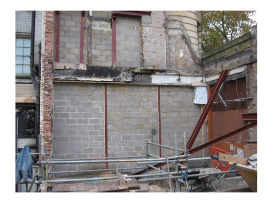
Photograph 2 Indicating existing steelwork and walls to rear of 8 - 10 Southampton Row -North east corner, including props to flank facade (taken prior to installation of felt and batten waterproofing)
