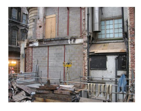
Photograph 1 Indicating existing steelwork and walls to rear of 8 - 10 Southampton Row - South east corner (taken prior to installation of felt and batten waterproofing)
