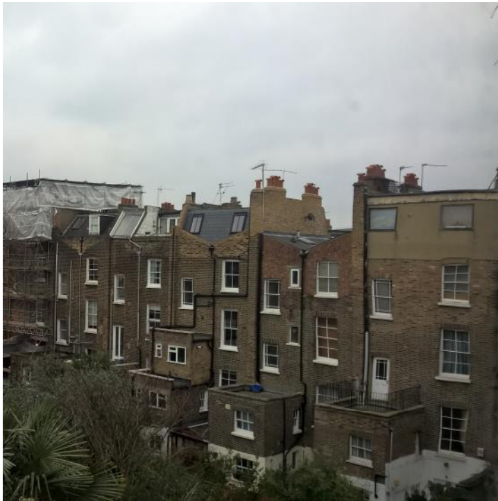
Rooftop extensions to the rear of the property
