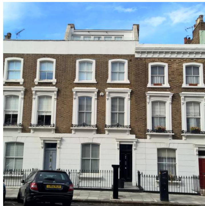
Rooftop extension to No. 18 Chalcot Road
