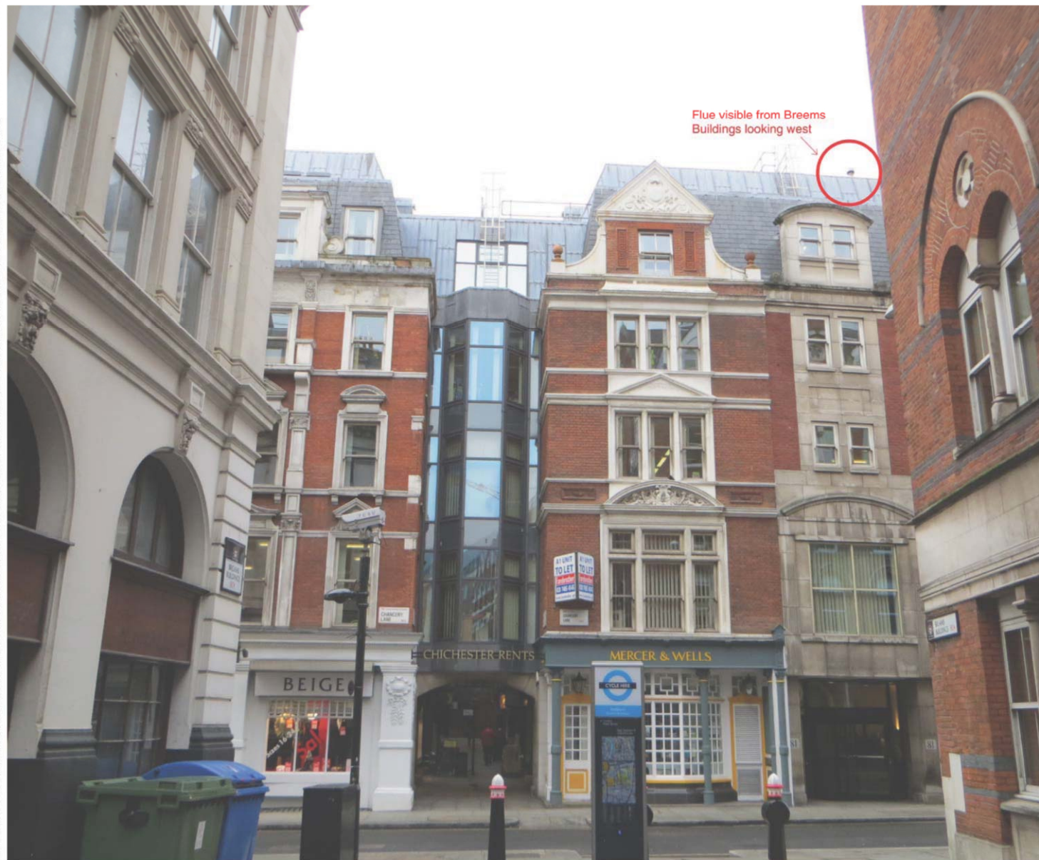
EXISTING VIEW 3 Breems Buildings looking West
