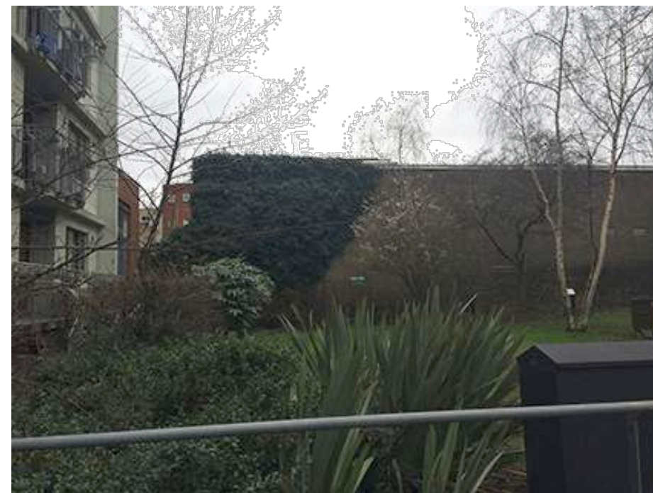
West Elevation - from Birkenhead Estate
