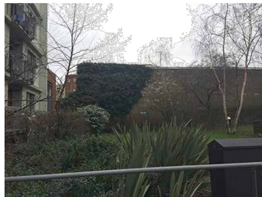
West Elevation - from Birkenhead Estate
