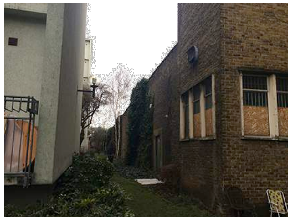
West Elevation - from Birkenhead Estate
