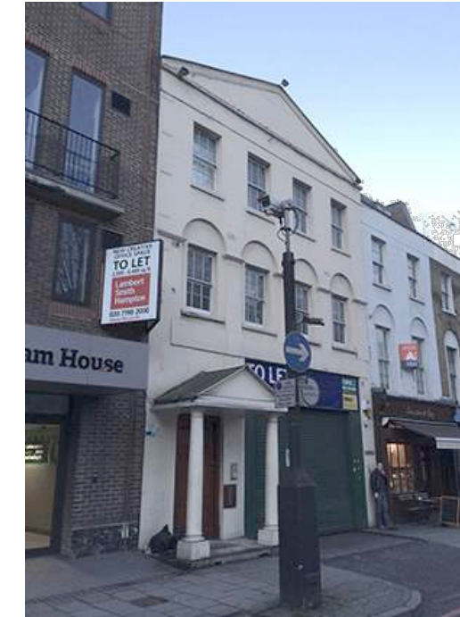
Gray's Inn Road entrance
