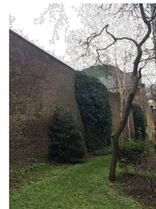
West Elevation - from Birkenhead Estate
