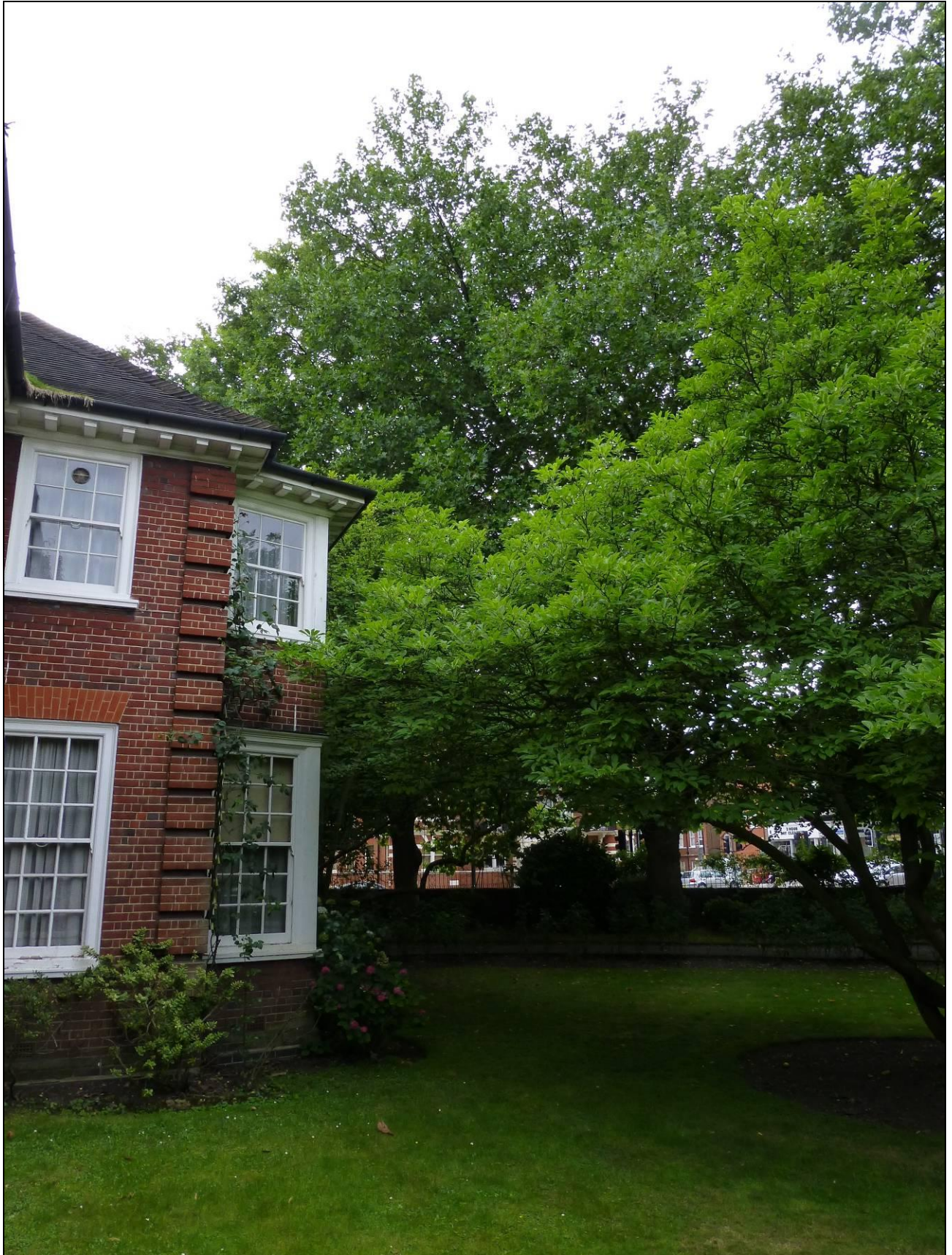
Photograph B - Showing the existing relationship between the building and trees.
