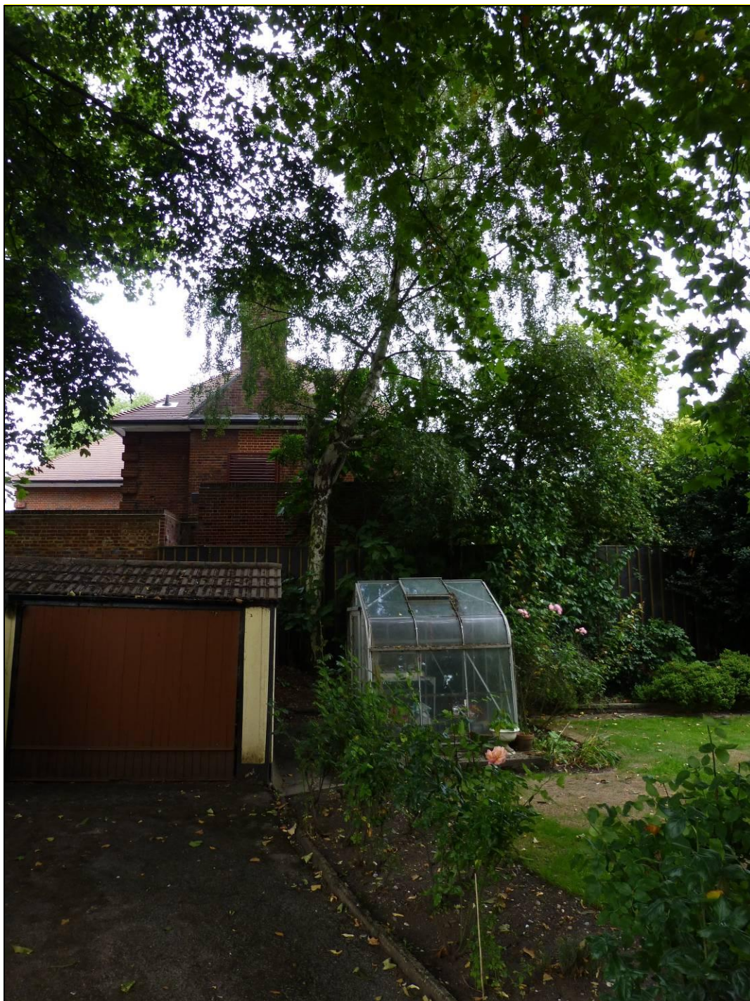
Photograph D - Looking towards the existing garage from the tarmac driveway.
