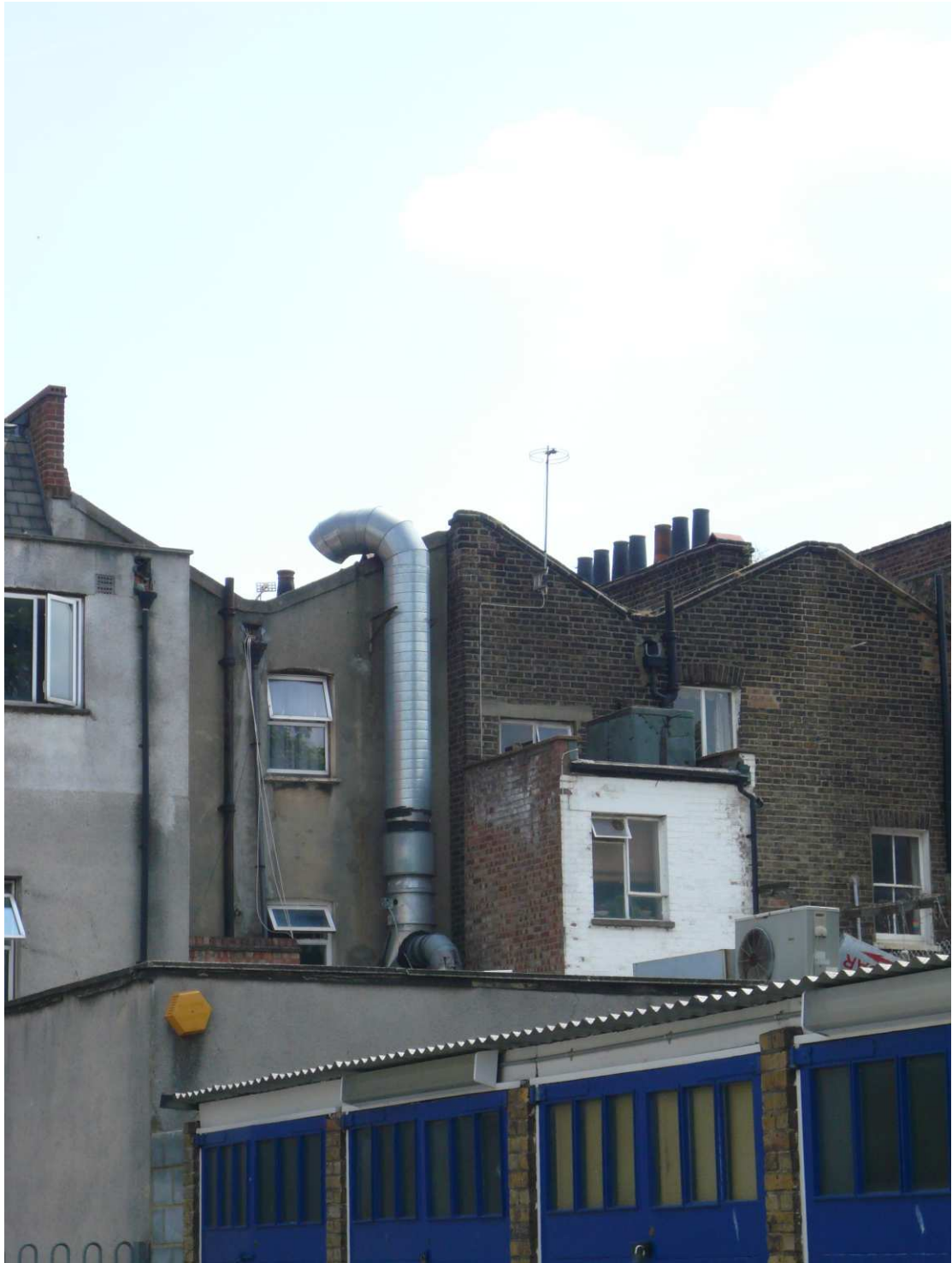
VIEW OF THE REAR OF PROPERTY
