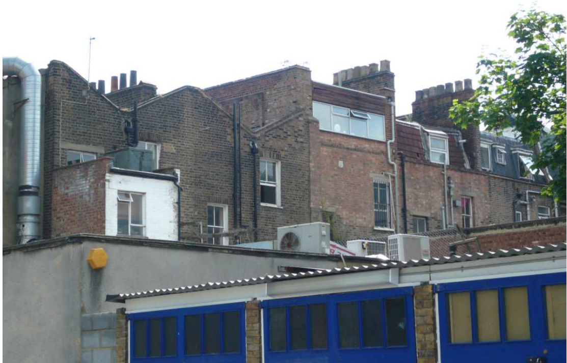
VIEW OF THE REAR OF PROPERTIES no. 67-59
