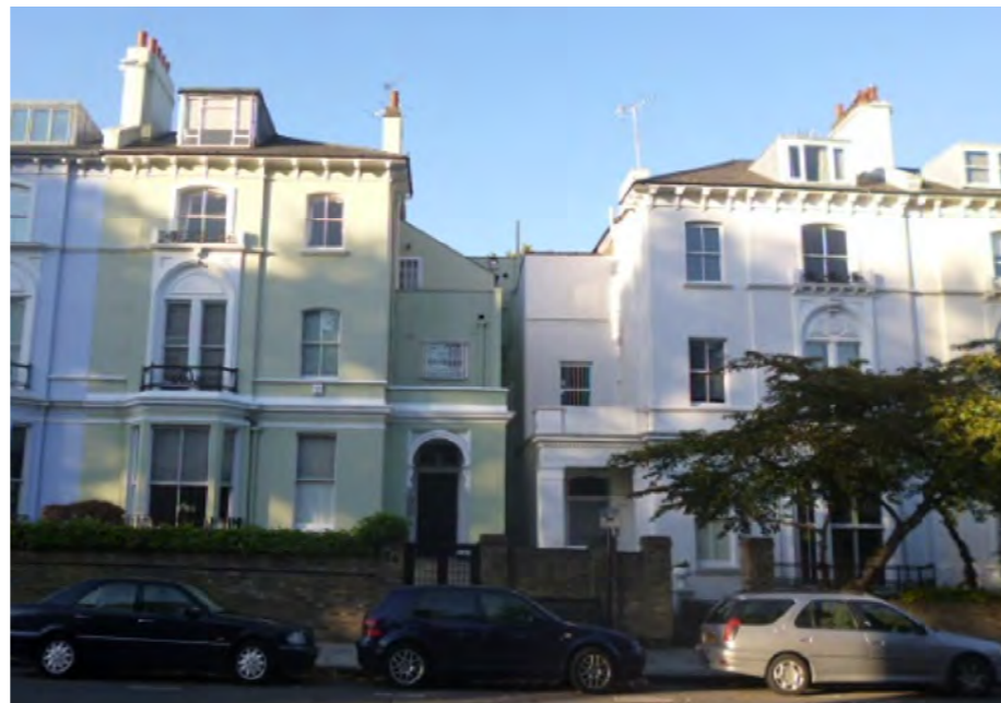
⑤ FRONT VIEW 54 REGENT'S PARK ROAD WITH No.52 ON RIGHT
