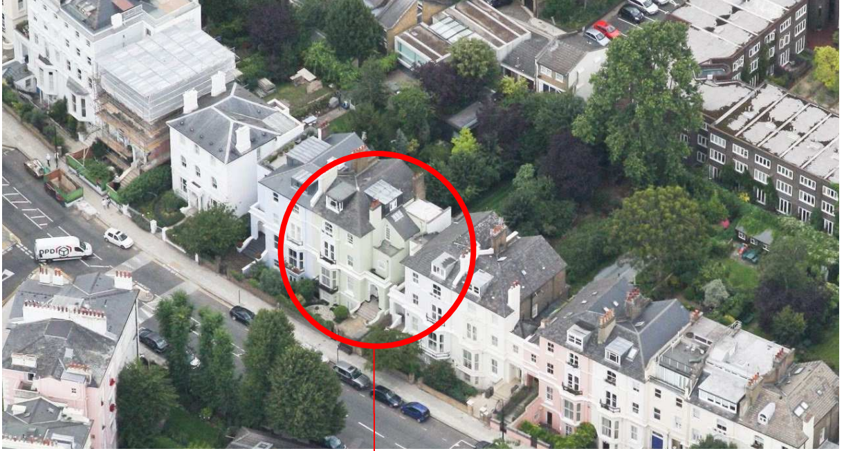
Aerial Photograph 1: Regent's Park Road from South (© Bing Maps).
