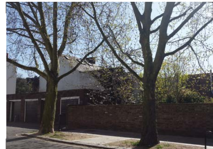
Side / rear elevations from Jeffrey's Street
