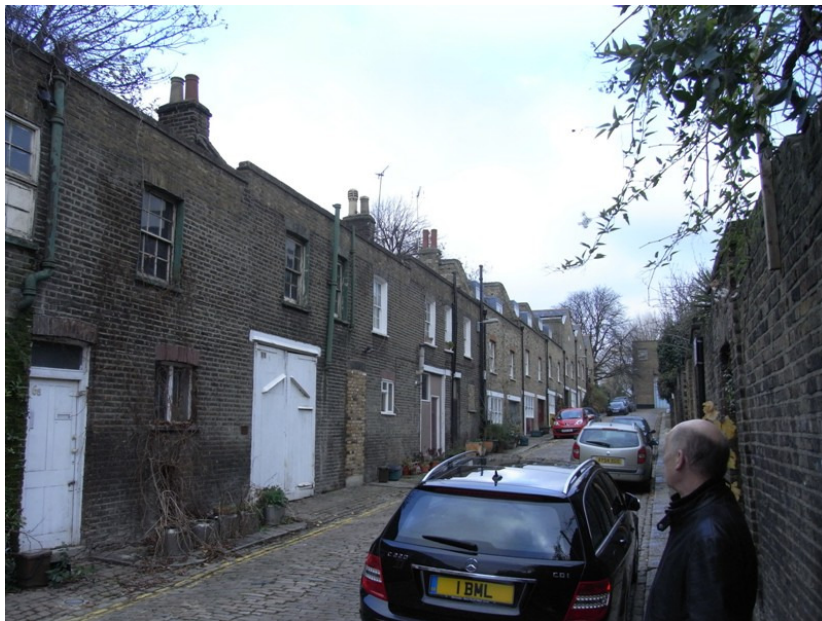
6 & 7 Railey Mews looking up past 8 Railey Mews to mansard roofing to 9, 10 and 11 Railey Mews which set precedent for this proposal.
