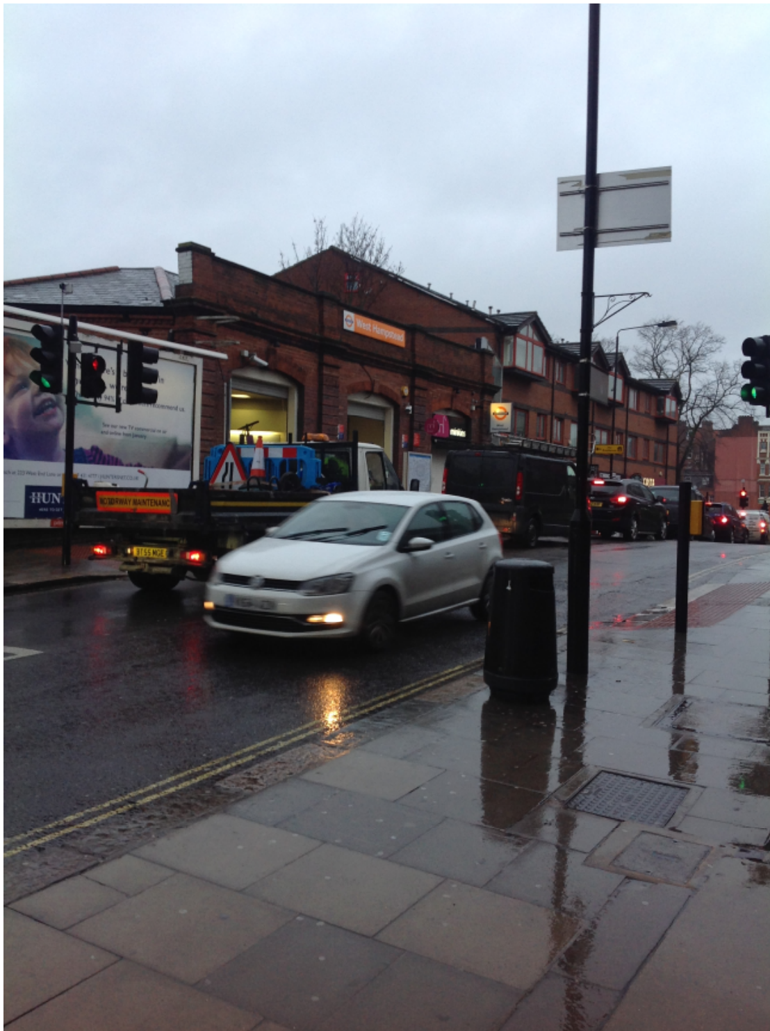
Photo 2: View of station from the eastern side of the road
