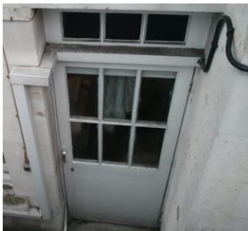
Existing Panel above door to be replaced with louvre.
