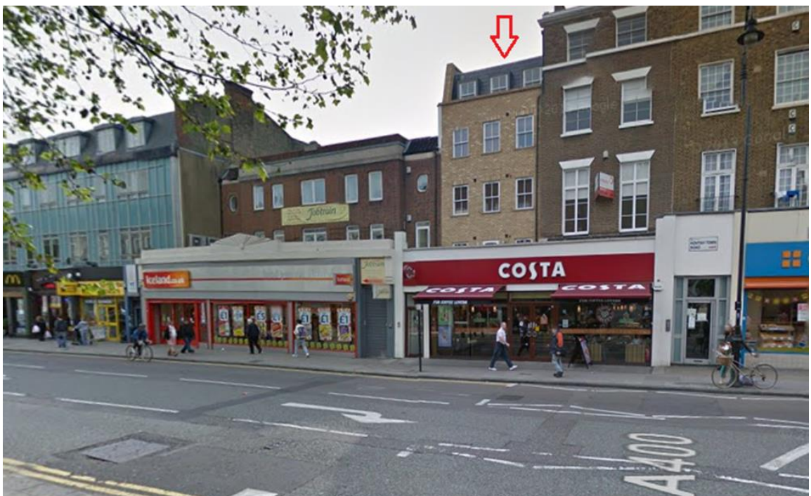
Figure 2: View of 309 Kentish Town Road
