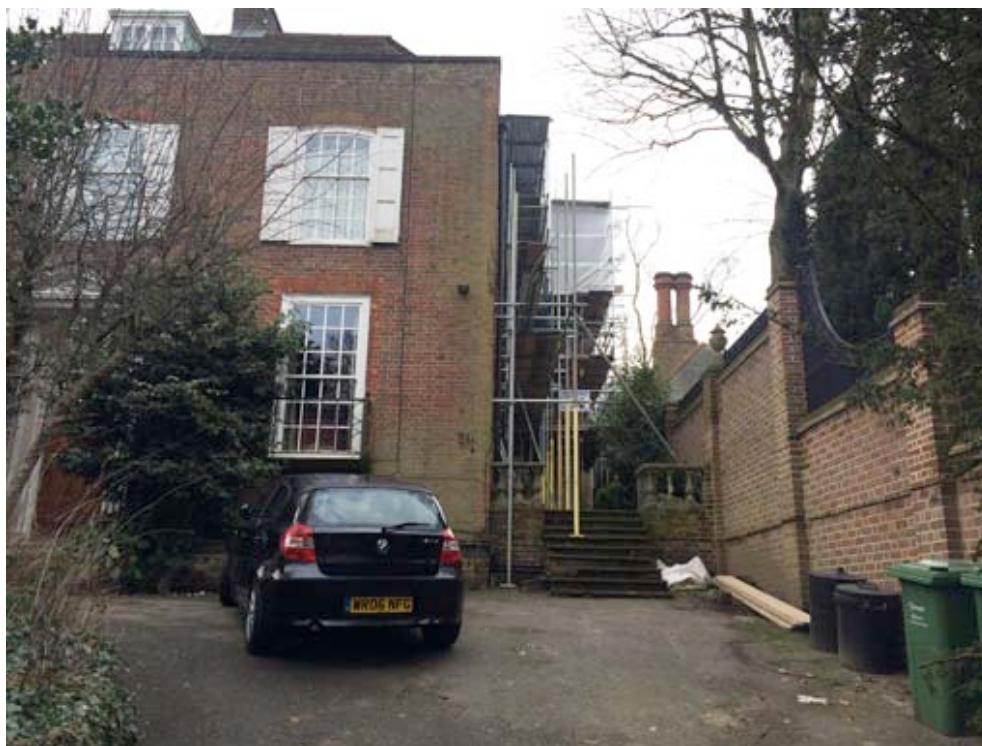
Approach to No.21B West Heath Rd.
