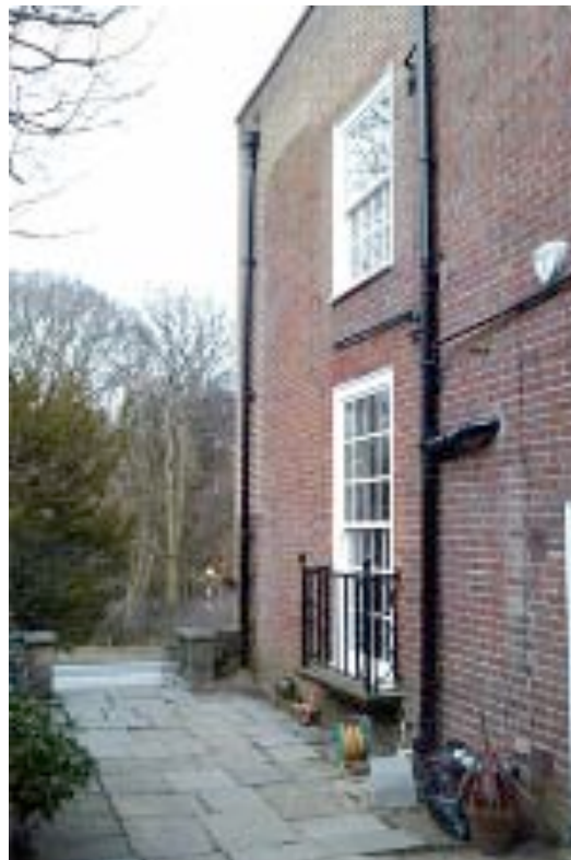
View from side passage towards front
