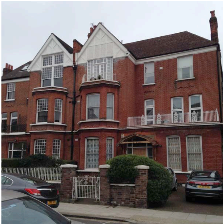
Photo 1 – the south elevation of No 46 showing a mix of different windows
