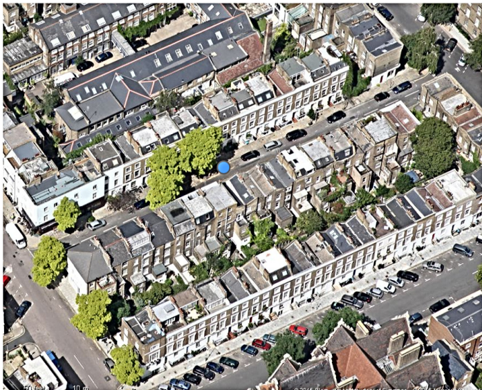
Aerial view of Edis Street showing the variety of roof extensions.
