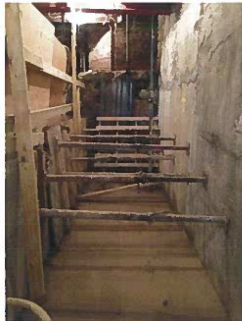
Image of Stage 3 on Site
