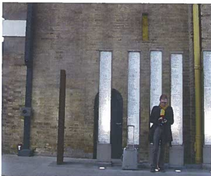
Photo showing the door to the Clock Tower behind the war memorial
