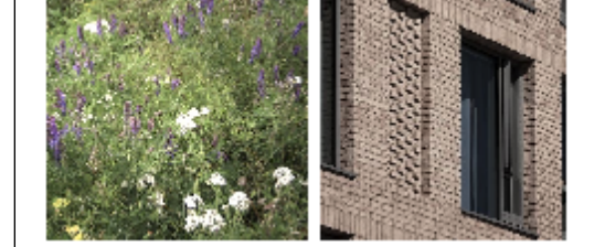
Integrated Soft Landscaping throughout. Bio-Diverse & Sedum roofs. Areas of relief in the brick work and changes in bond & colour
