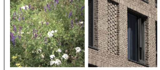
Integrated Soil Landscaping Throughout. Bio-Diverse Sedum roofs. Areas of relief in the brickwork and changes in bond & colour
