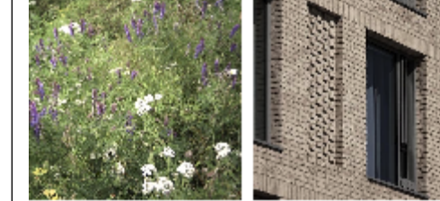
Integrated Soft Landscaping throughout. Bio-Diverse & Sedum roofs. Areas of relief in the brick work and changes in bond & colour.
