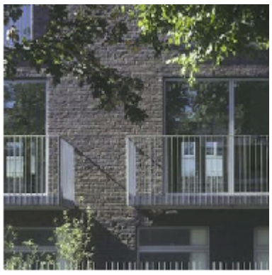
Projecting balconies - Flat steel section balustrades. Architect: Tony Fretton
