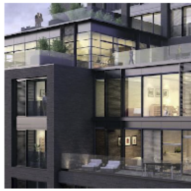
Upper storey flats glazed to the north and south with private terraces.
