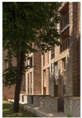
Varying reveals to articulate forms and massing. Architect: Panter Hudspith
