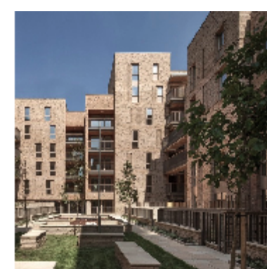
Varying reveals to articulate forms and massing. Architect: Panter Hudspith
