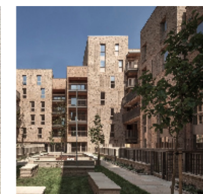
Varying reveals to articulate forms and massing. Architect: Panter Hudspith
