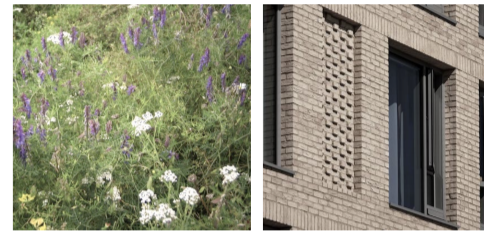
Integrated Soft Landscaping throughout. Bio-Diverse & Sedum roofs. Areas of relief in the brick work and changes in bond & colour
