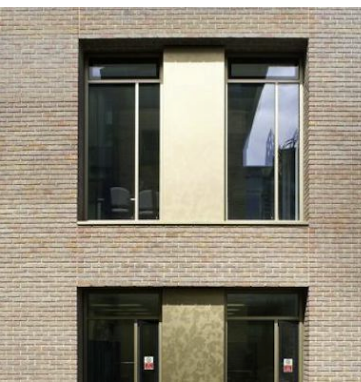
Deep brick reveals with aluminium windows & panels. Architect: Hawkins/Brown
