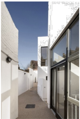
Subservient mass to the rear of an existing terrace. Architect: Peter Barber
