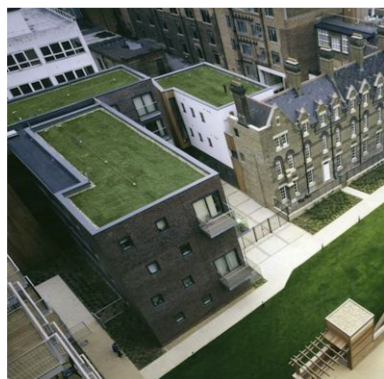
Green roofs provide visual amenity to both neighbouring and new occupants. Architect: HawkinsBrown
