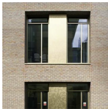
Deep brick reveals with aluminium windows & panels. Architect: Hawkins/Brown
