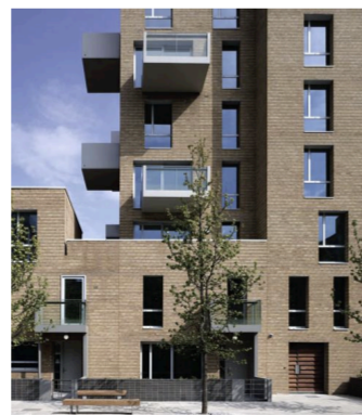
Stepping & recessed massing Architect: Allies and Morrison
