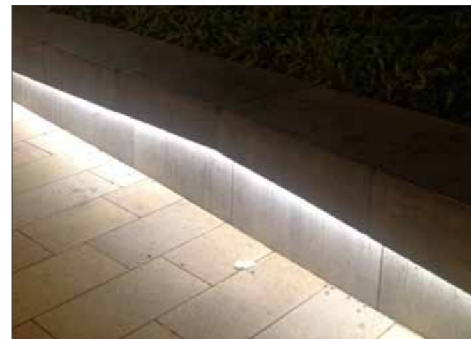
Integral lighting strips to the raised planters
