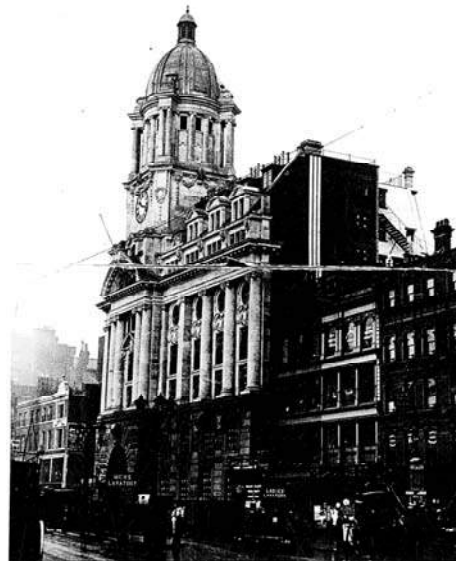
Phase I complete, 1913.
