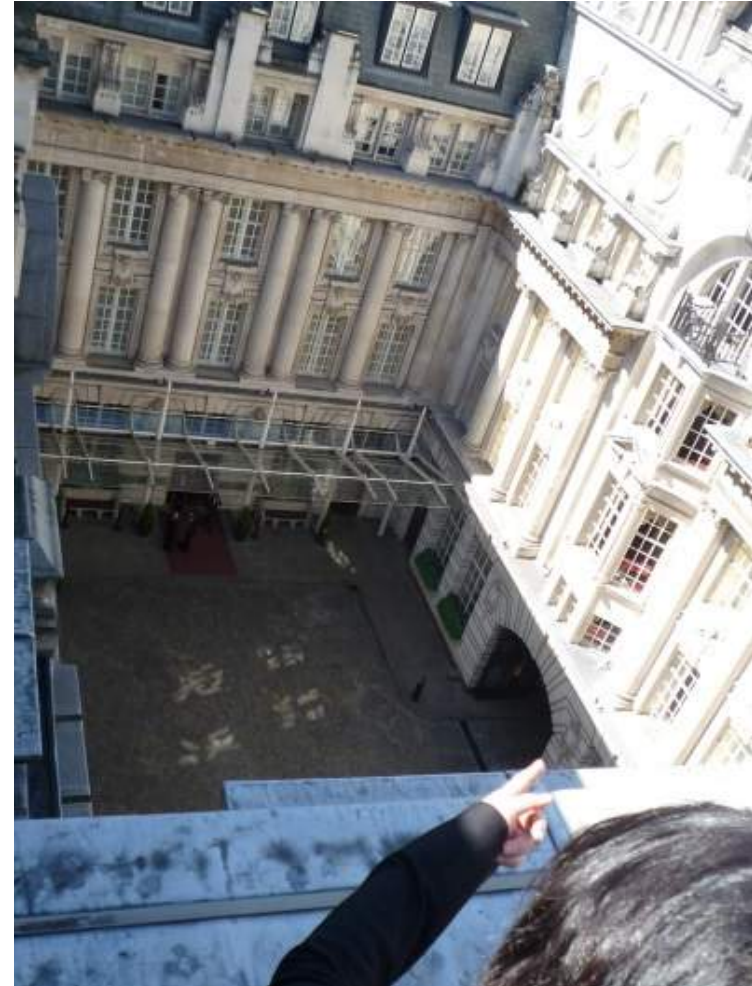
The Courtyard with glazed screen installed in the TP Bennett Scheme prior to the EPR 2013 scheme.
