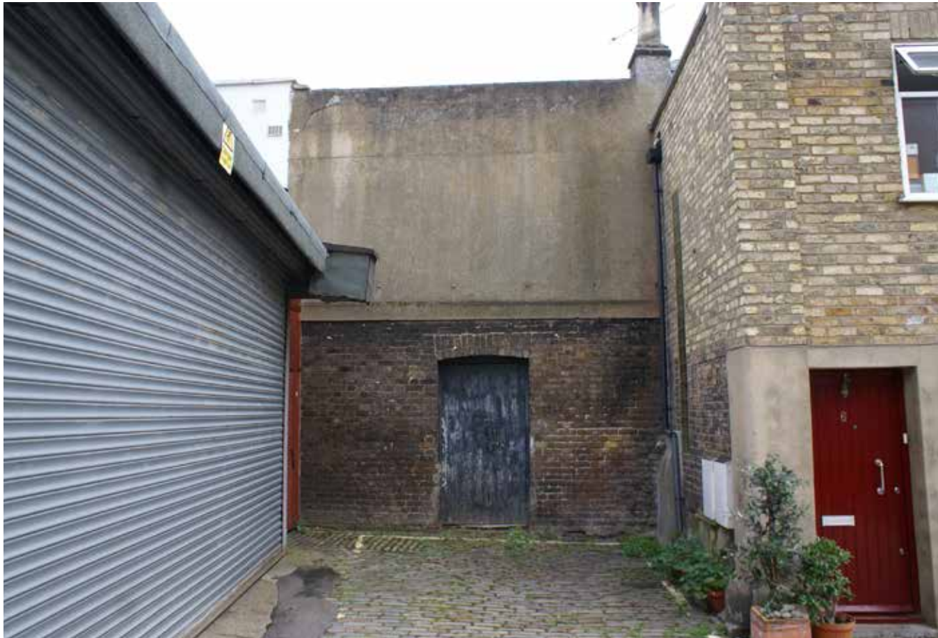
Above: Fig. 4 - Existing garage and adjacent site buildings
