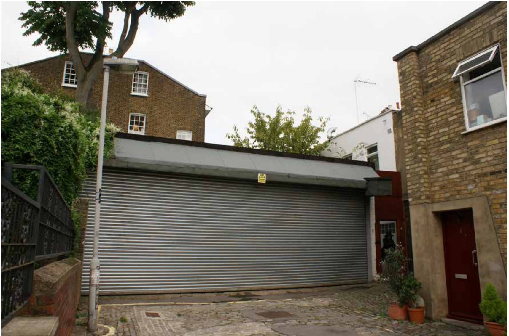
Fig. 3 - The site currently comprises an empty single storey private garage with a large rolling shutter door and space for up to three vehicles. It sits as a stand alone building at the end of the mews, with a separate appearance to the rest of the buildings. The existing garage covers the entire footprint of the site.
