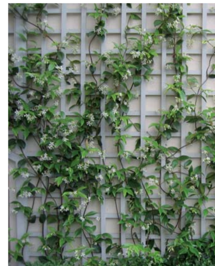
Trelliswork to walls
