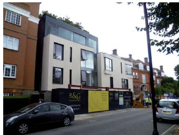
VIEW 3 - 5 NUTLEY TERRACE (UNDER CONSTRUCTION)
