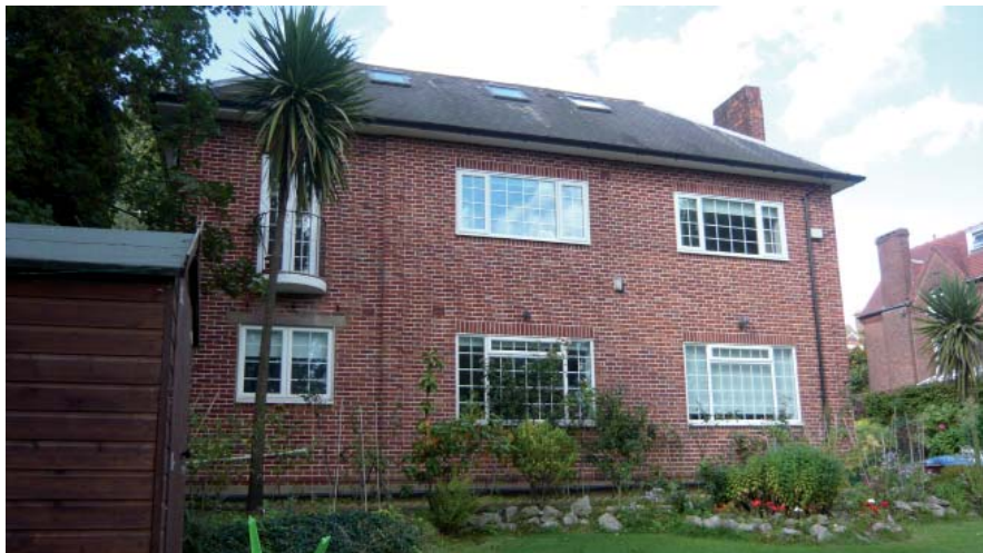
VIEW 3 - NO.6 VIEW FROM REAR GARDEN
