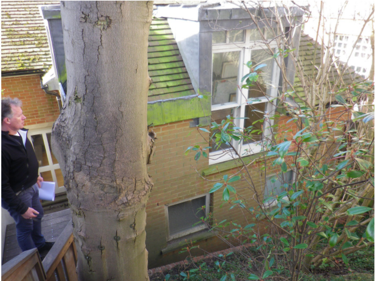
Existing Dormer window and 2 lower windows
