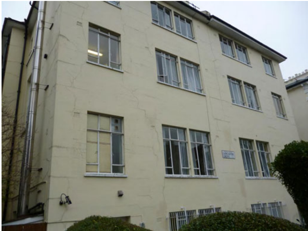
Figure 1: View of the building from Lancaster Grove.
