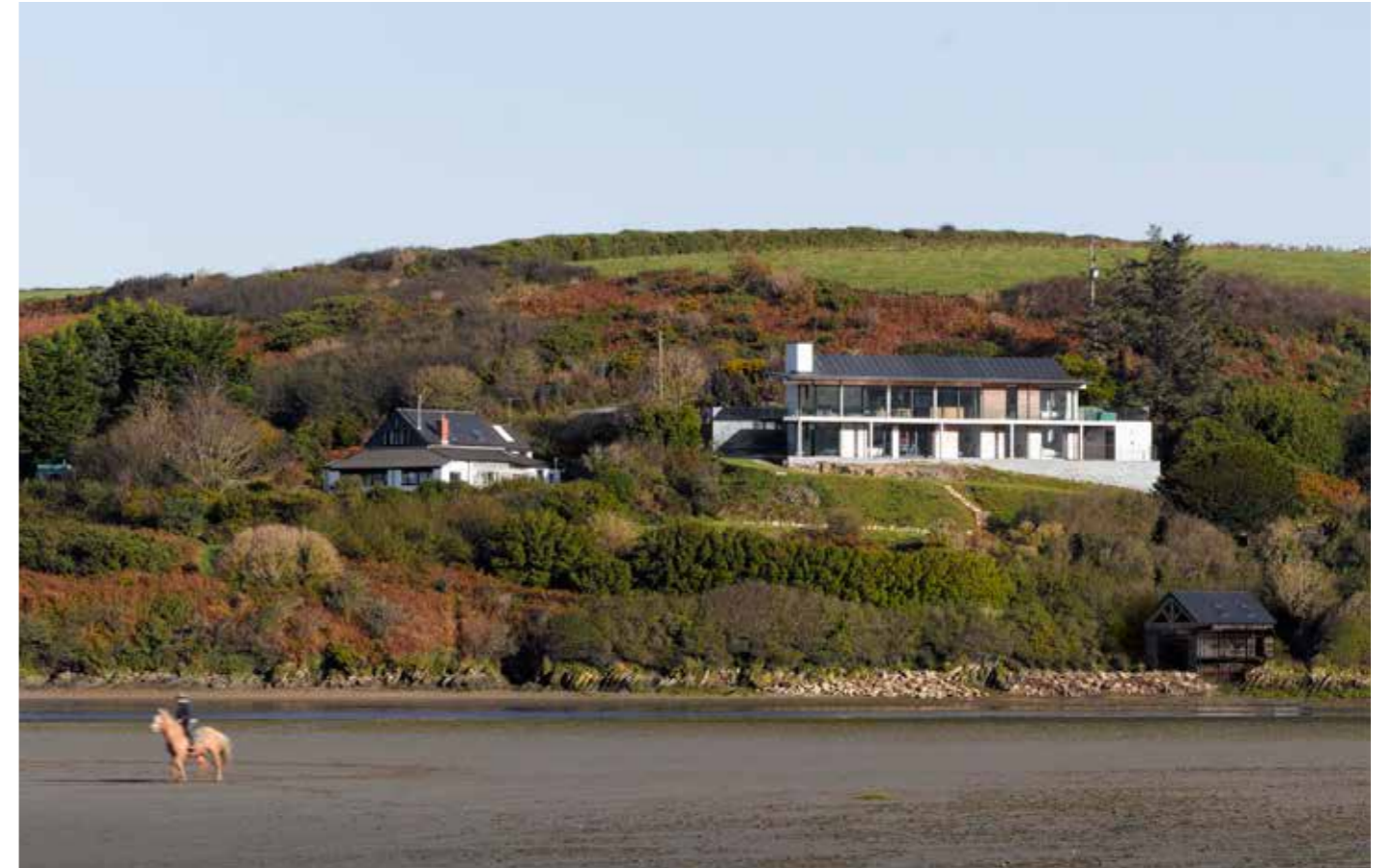
Trewarren House, West Wales. RIBA Award 2013 and Gold Medal Award for Architecture in Wales 2013
